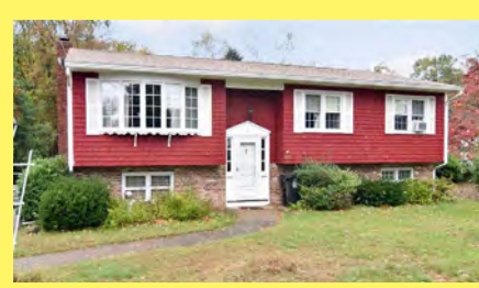
SWANSEA Raised Ranch $329.900
